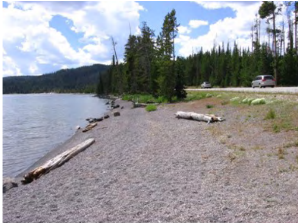
Fig. 1: These images are from the beach compartment just north of the Potts Springs Thermal Basin. A) Non-engineered shore segment. Note the wide, gently sloping beach and its proximity to the road. B) Engineered segment. Notice the rip-rap along the length of the shoreface and the complete lack of a dry beach.
