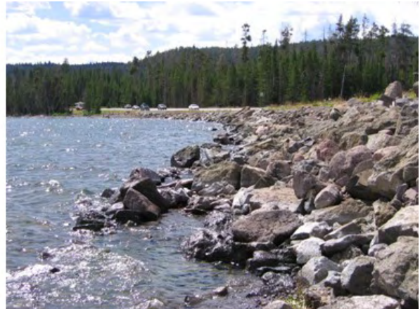
Fig. 1: These images are from the beach compartment just north of the Potts Springs Thermal Basin. A) Non-engineered shore segment. Note the wide, gently sloping beach and its proximity to the road. B) Engineered segment. Notice the rip-rap along the length of the shoreface and the complete lack of a dry beach.
